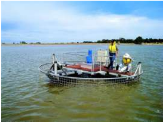
Figure 4-2 Mechanical mixer (left) and aerator (right) at Myponga Reservoir
