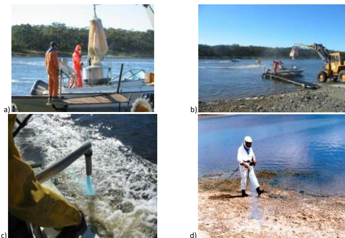
Figure 4-5 Copper sulphate dosing of a reservoir (a-c) and benthic cyanobacteria after reservoir draw-down d)
