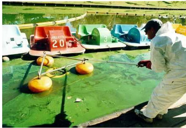
Figure 4-3 The use of a skimmer to remove surface scum in a recreational lake in South Australia. Toxic material was collected and disposed to sewer
